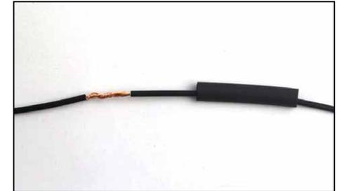
2. Twist wires together and make sure the sleeve is kept away from any heat source
